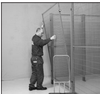
Panels are dismantled using an Allen key.
